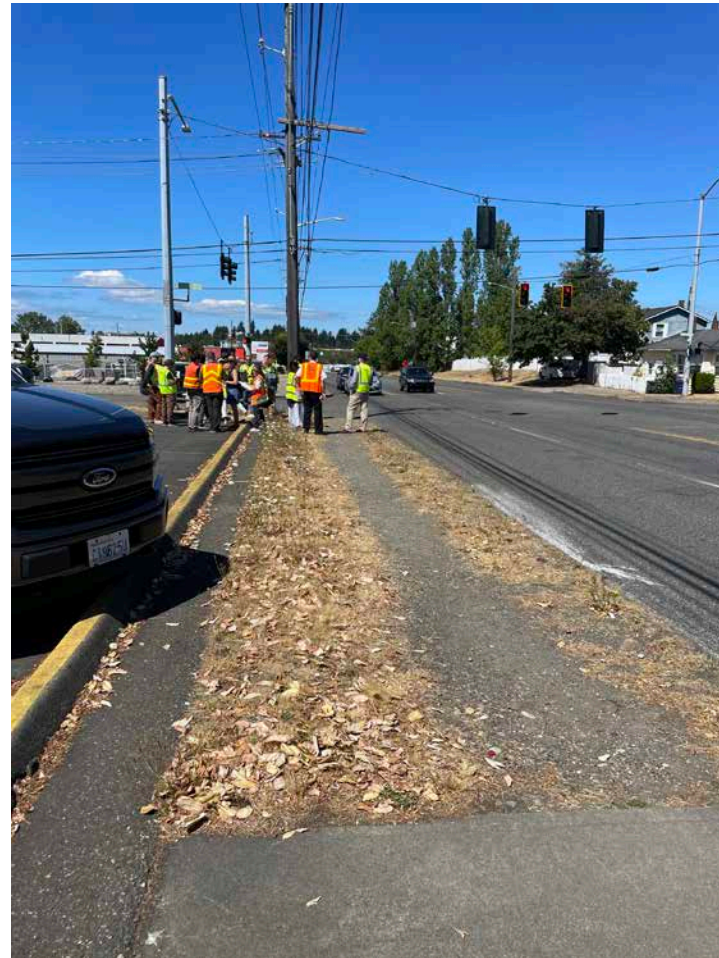
Missing link sidewalk south of S 36 th St
