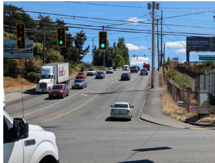
Steep slope south of S Tacoma Way
