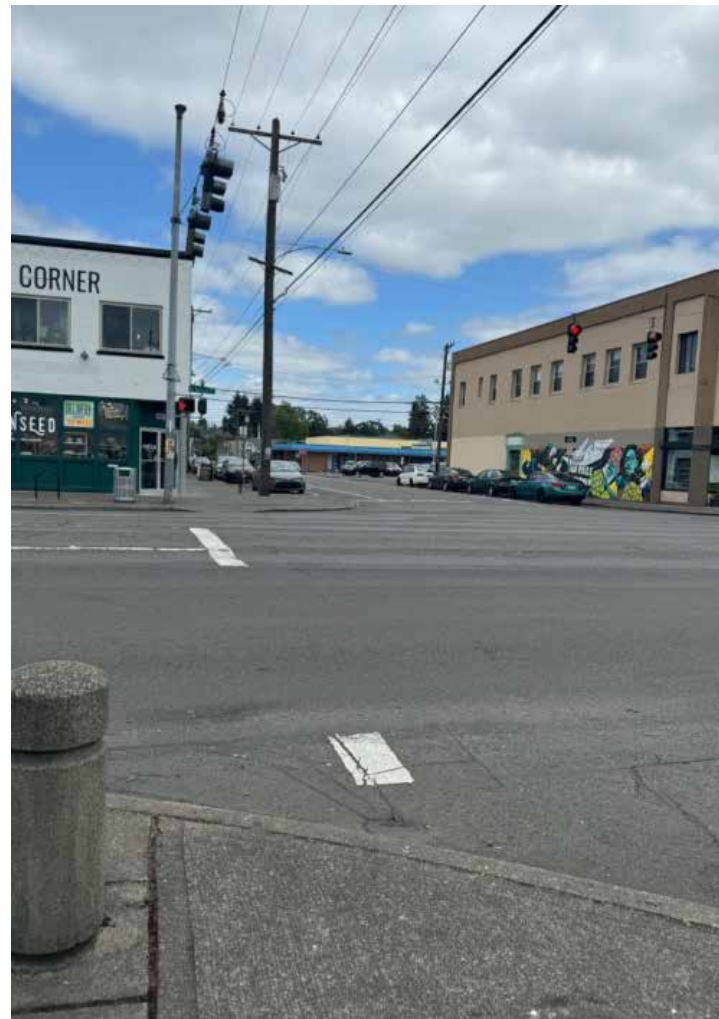
No marked crosswalks at S Tacoma Way-S 54 th St intersection
