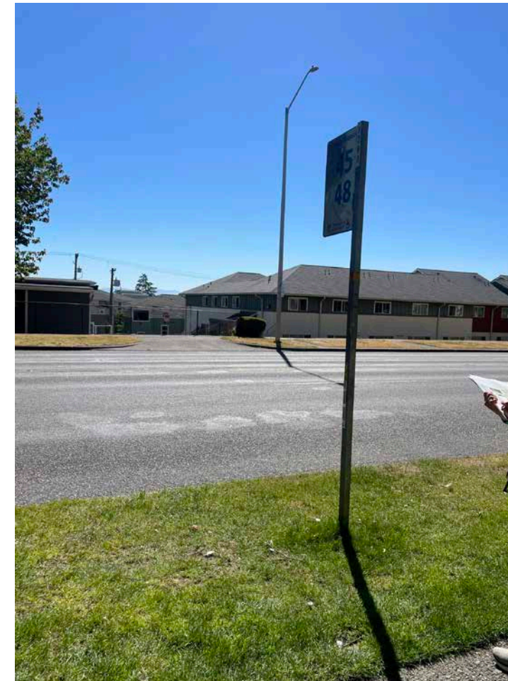
Bus stop without front or rear pads at S 17 th St
