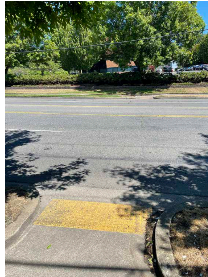
Curb ramp at least 20 feet south of S 43 rd St intersection
