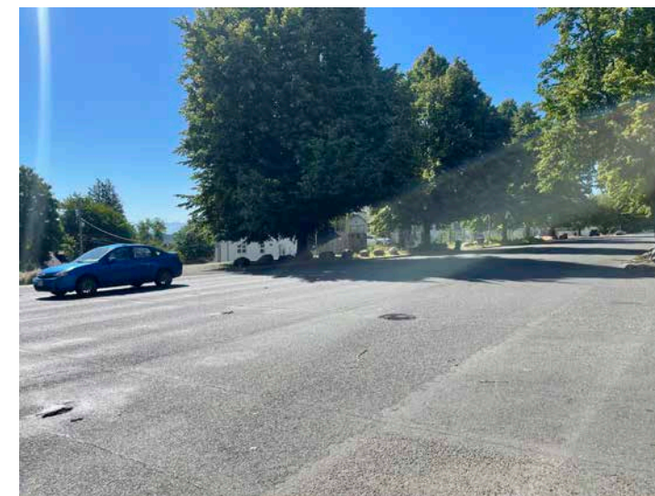
Large uncontrolled and unmarked intersection at S 16 th St
